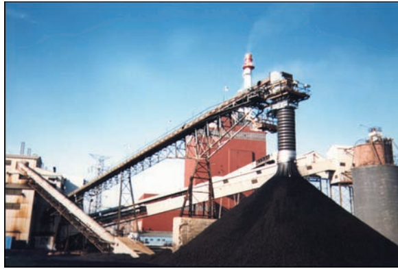
Dust free coal stockpiling.
