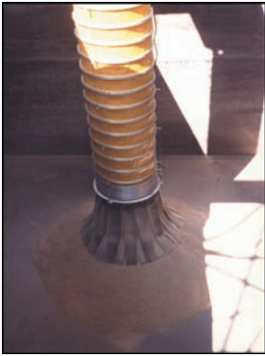
Dust free grain loading into barges.
