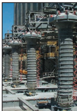
Ship loading spouts utilizing compact filter modules
