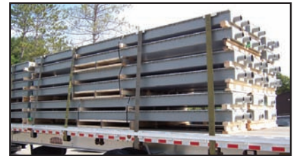
Aerated troughs for dome floor installation.
