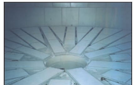
30'-0" diameter fully aerated flat bottom silo using aeration troughs.
