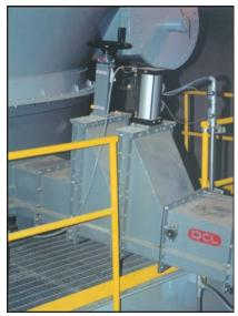
Vertical manual and pneumatic slide gate valve.
