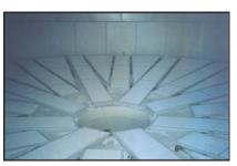
30'-0" diameter fully aerated flat bottom silo using aeration troughs.
